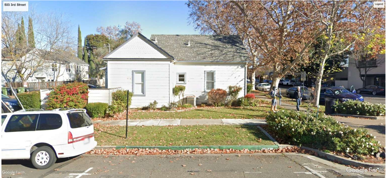
Figure 4 –503 3 rd street, side view (Google Earth 05/30/2023)
